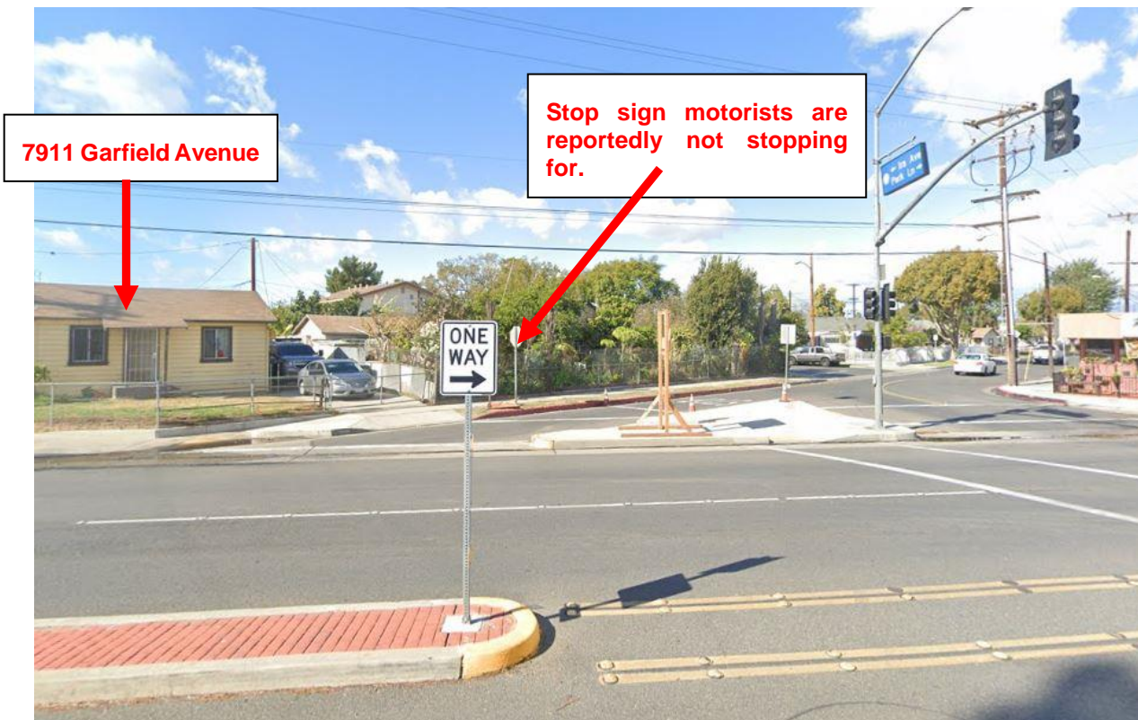
Figure 4 - Street View of 7911 Garfield Avenue at Ira Avenue Looking West
