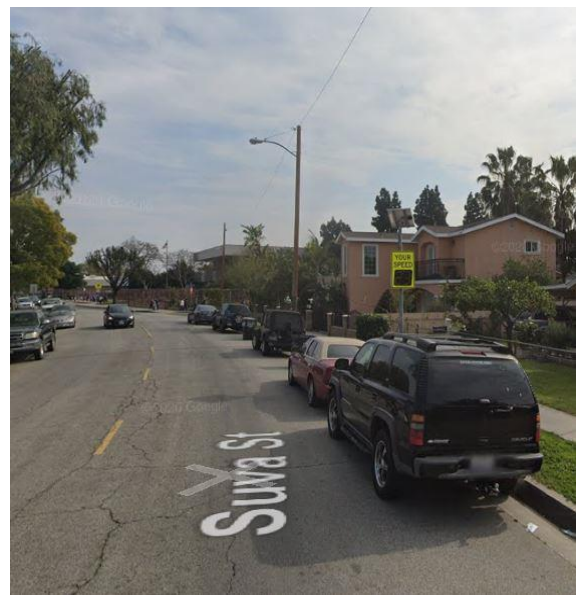
Figure 3 – Looking South on Suva by Loveland St.
