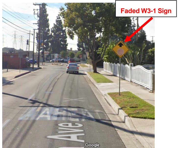
Figure 3 - Ira Ave. Looking South Faded W3-1 Sign
