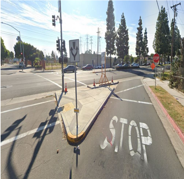
Figure 2 - Ira Ave. at Garfield Ave. Looking South
