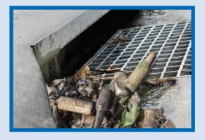
Thirty-nine pipe screens will be installed in the flood control catch basins that are within the City limits. The screens will retain debris until the basins are cleaned by City maintenance crews, who service them monthly.
